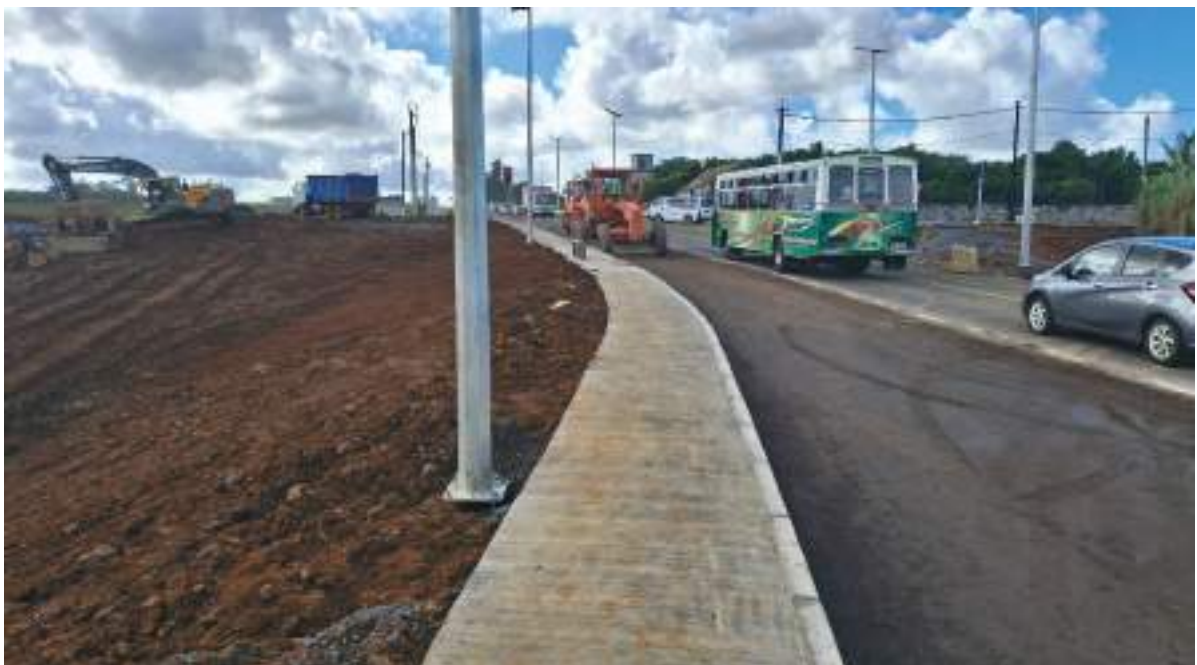
Figure 11: Upgrading of Savanne Road (A9) from La Flora to Tyack
