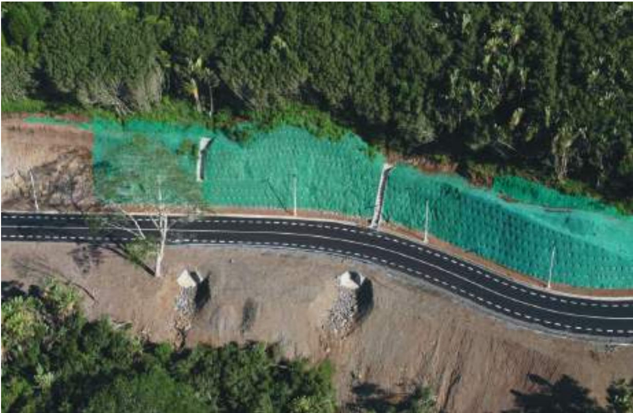
Figure 1: Stabilisation Works along B103 Road at Chamarel
