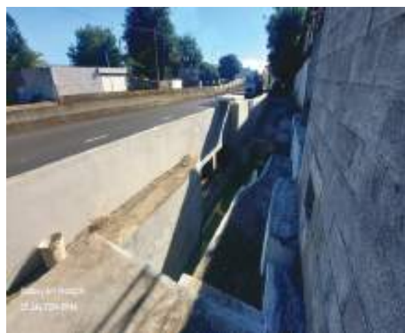
Figure 16: Road Conditions and Water Discharge After Completion of Works
