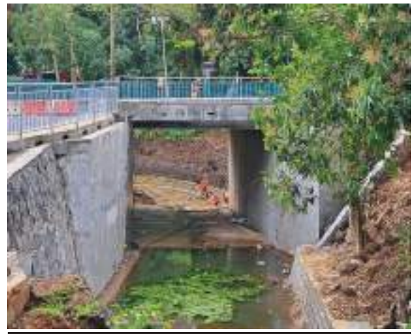
Figure 22: Road and Bridge Conditions Before Works
