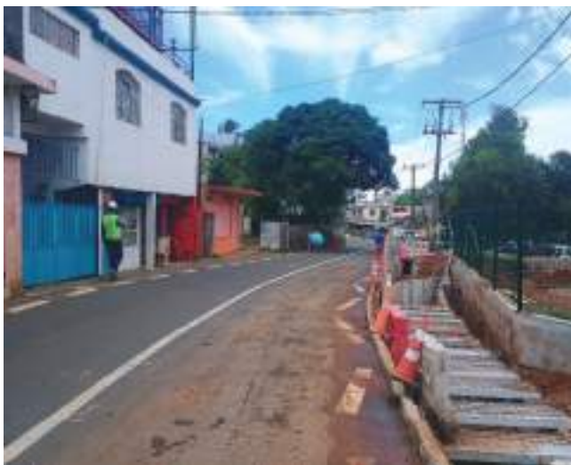
Figure 23: Road Condition Before Work
