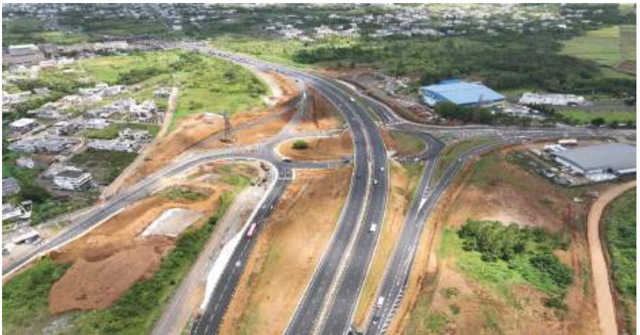
Figure 4: Construction of Flyover at Wooton
