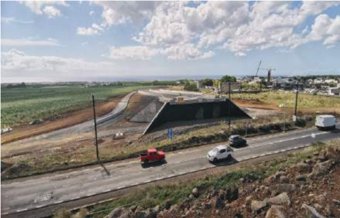
Figure 8: Construction of Flic-en-Flic Bypass from Xavier to Pierrefonds (Phase 3)
