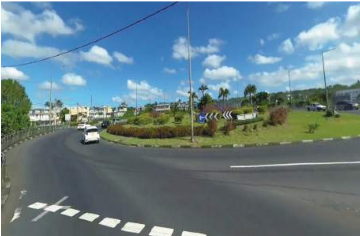
Figure14: Flyover at Camp Fouquereaux
