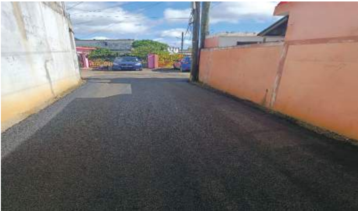
Figure 25: Resurfacing of chemin Rail at Circonstance
