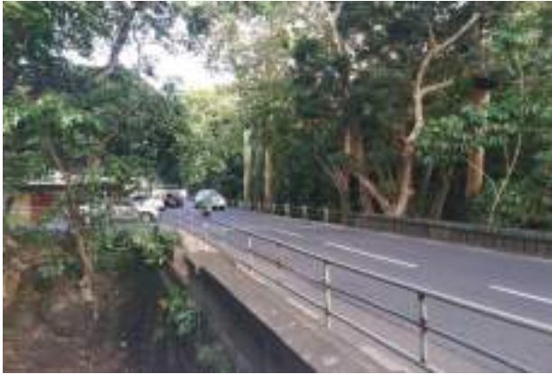
Figure 19: Road and Bridge Conditions After Works
