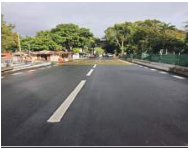
Figure 21: Road and Bridge Conditions Before Works
