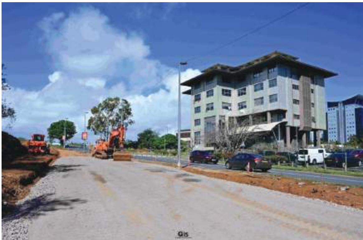
Figure 9: Upgrading of Julius Nyerere Avenue & Construction of B1-M1 Link Road
