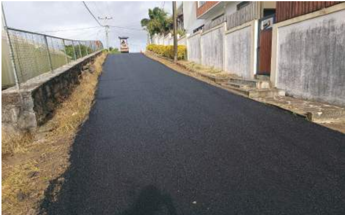
Figure 26: Resurfacing of Beelur Lane at Nouvelle Decouverte
