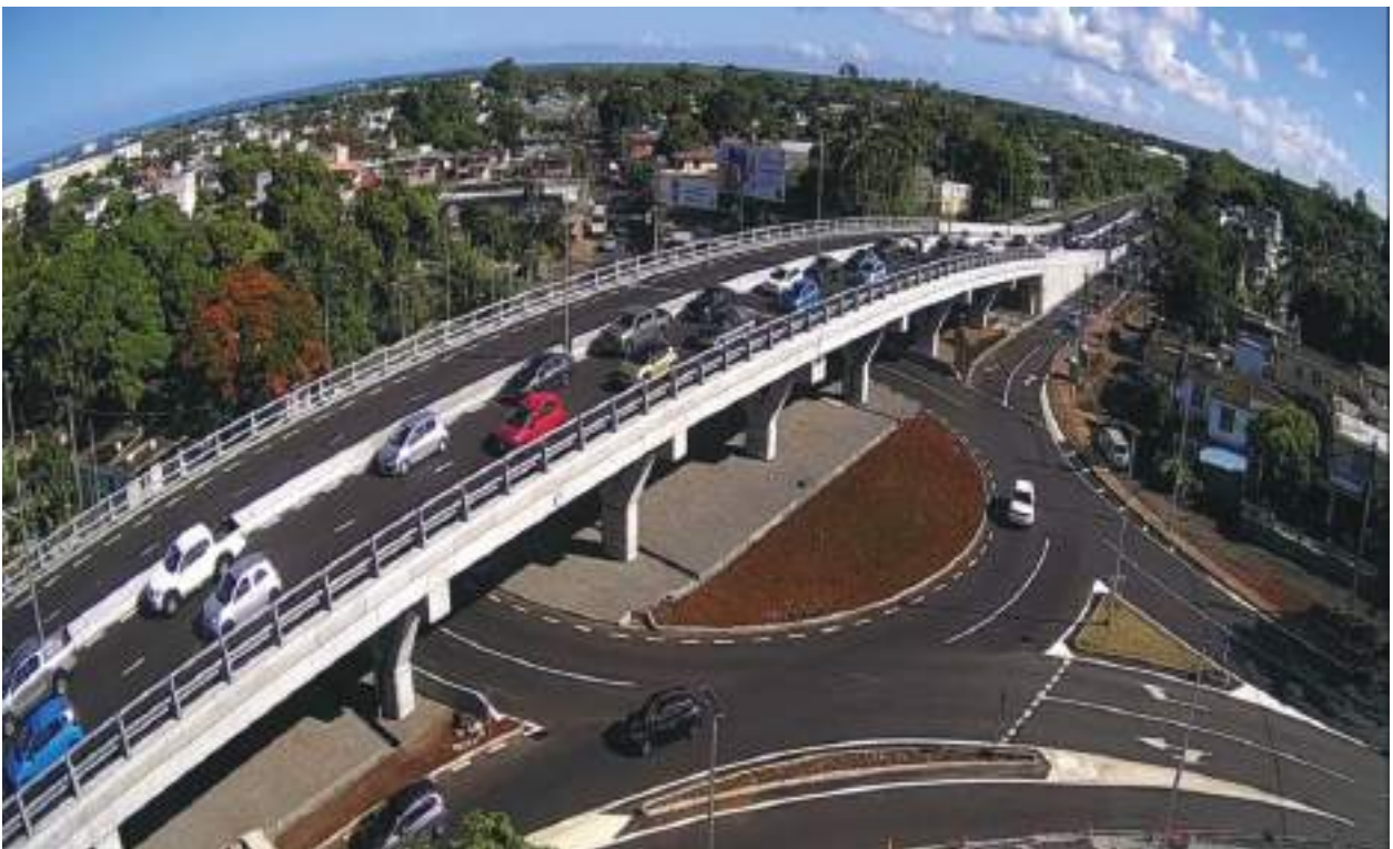
Figure 6: Construction of Flyover at Terre Rouge on Motorway M2
