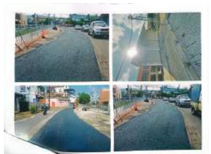
Figure 24: Road Condition After Work
