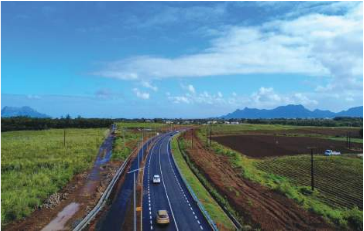
Figure 5: Construction of Hermitage Bypass
