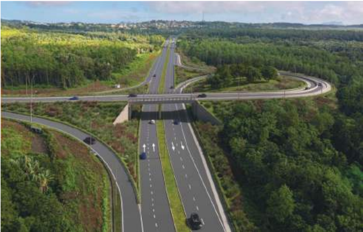
Figure 2: Construction of a Flyover on Motorway M1 at La Vigie
