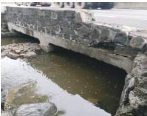
Figure 15: Road Condition and Water Discharge Before completion of works
