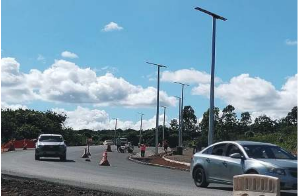
Figure 10: Upgrading of Part of Hollyrood Road
