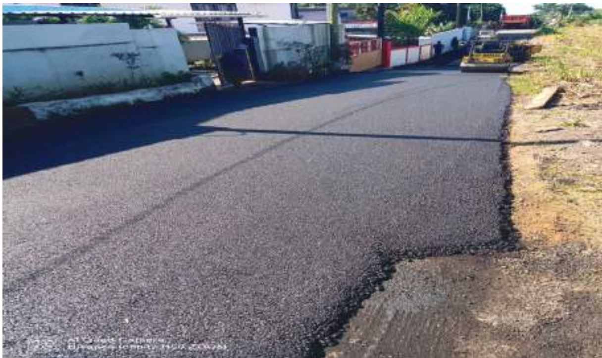
Figure 27: Resurfacing of School Lane at Petite Julie
