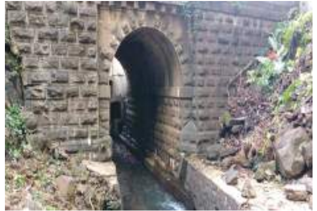
Figure 20: Road and Bridge Conditions After Works
