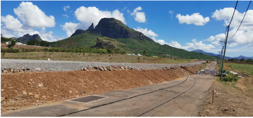
Plate 8: Layout of crusher run completed at Section 2
