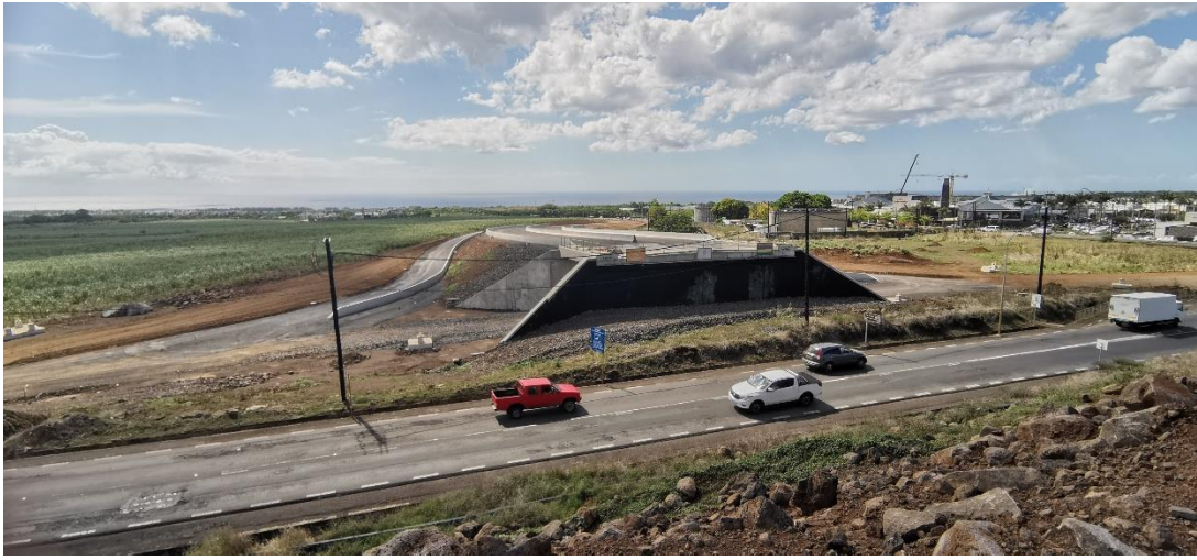
Plate 2: Underpass F completed at proposed grade separated junction at Cascavelle
