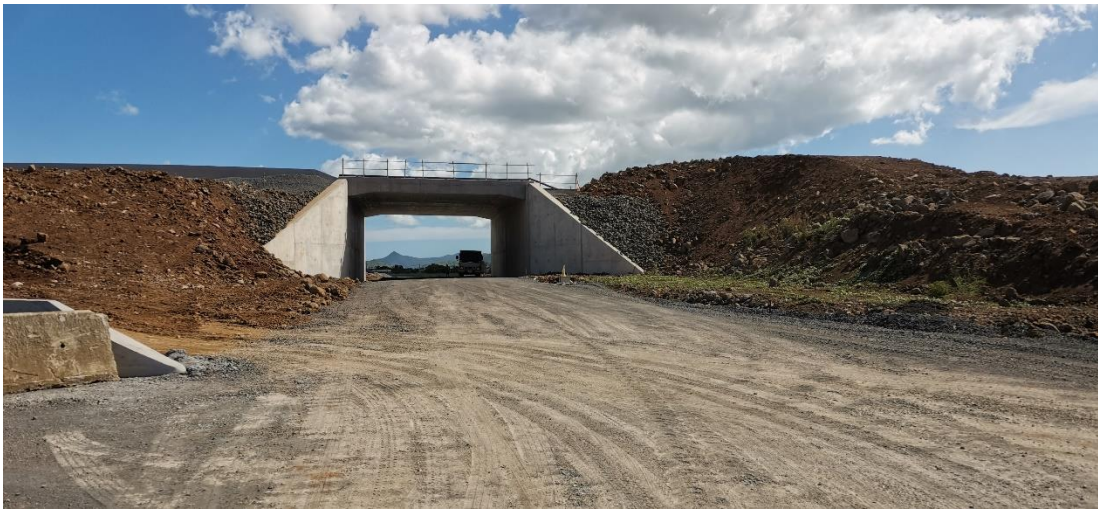
Plate 3: Underpass G completed at proposed grade separated junction at Cascavelle
