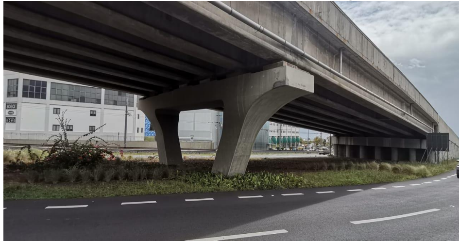
Piers under flyover (6 Nos.)
