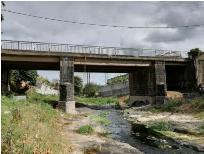
Picture 1: Stone Piers and retaining wall
