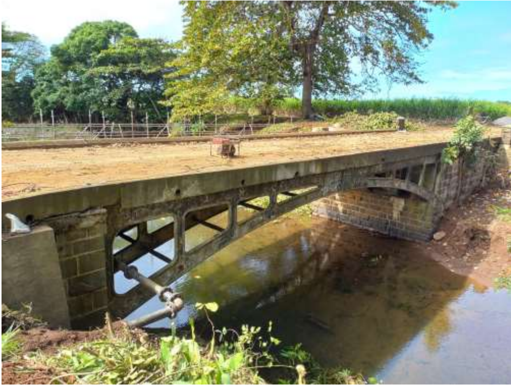
Fig 4: Preparation for Demolition of Existing Bridge
