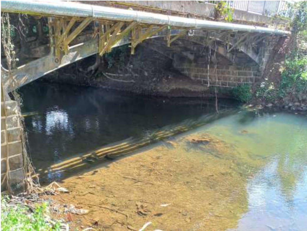
Fig 2: Existing Bridge view
