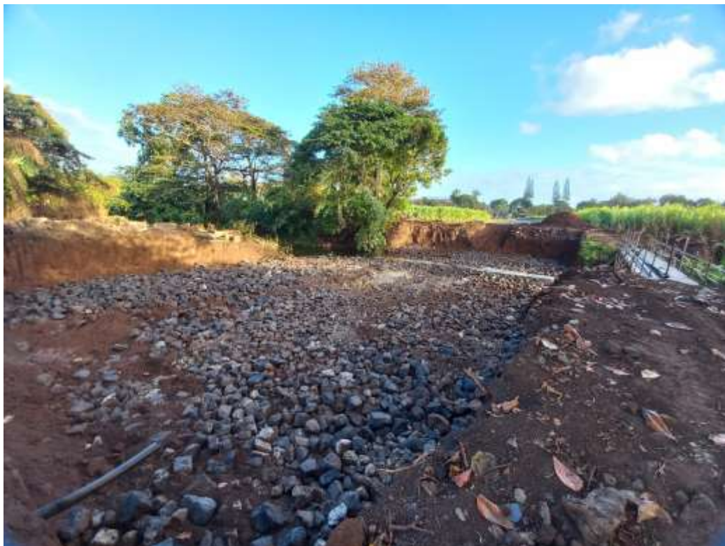
Fig 5: After demolition of Existing Bridge
