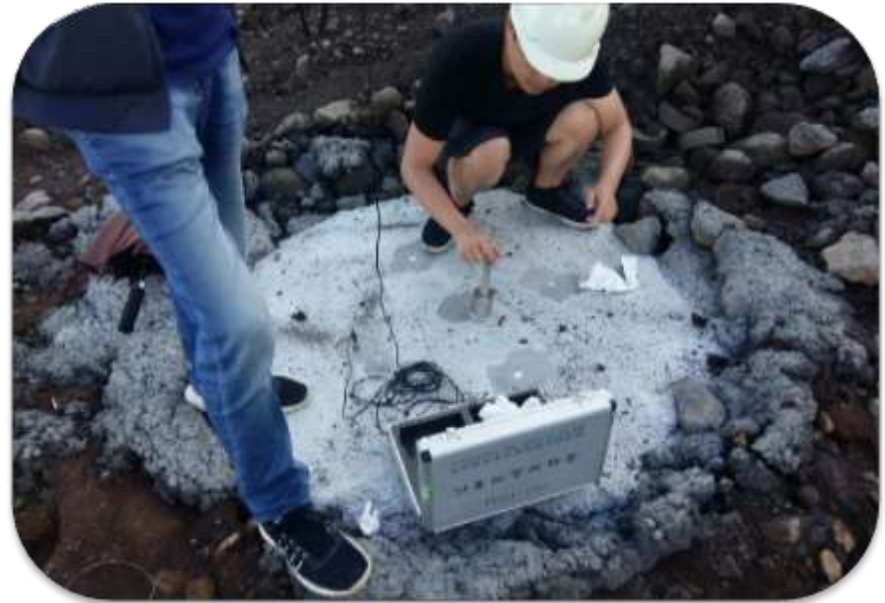
LOW STRAIN PILE INTEGRITY TEST
