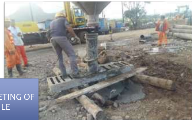
INSTALLATION OF CASING
