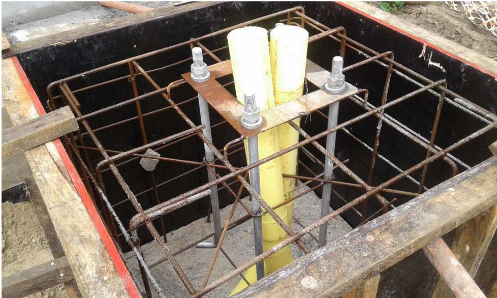
Figure 22: Reinforcement of streetlighting base
