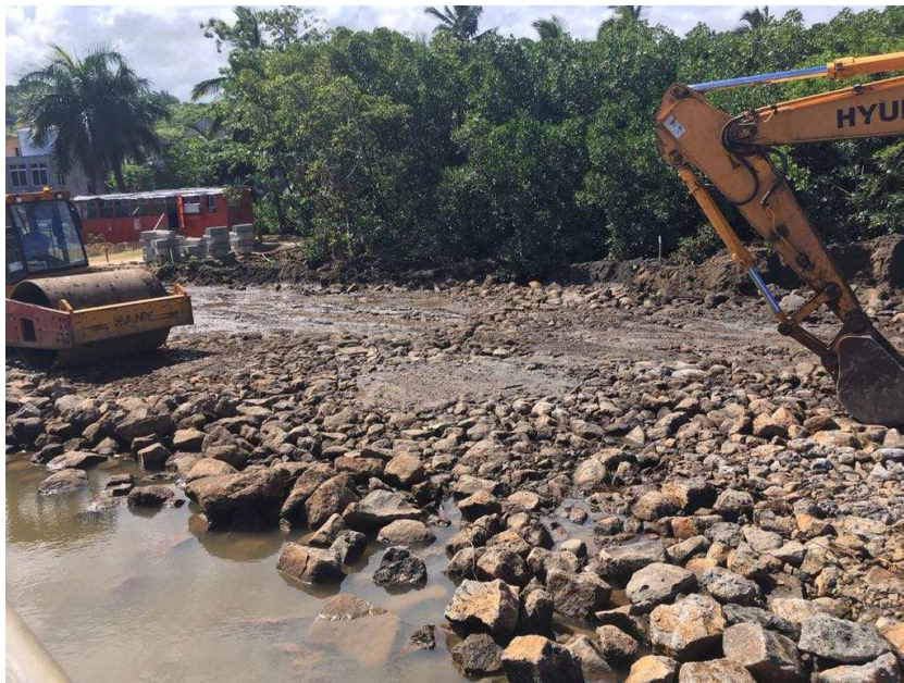
Figure 12: Rock filling followed by compaction by 18 ton roller
