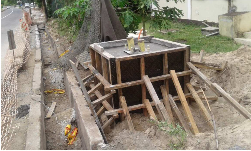
Figure 23: Casting of streetlighting base
