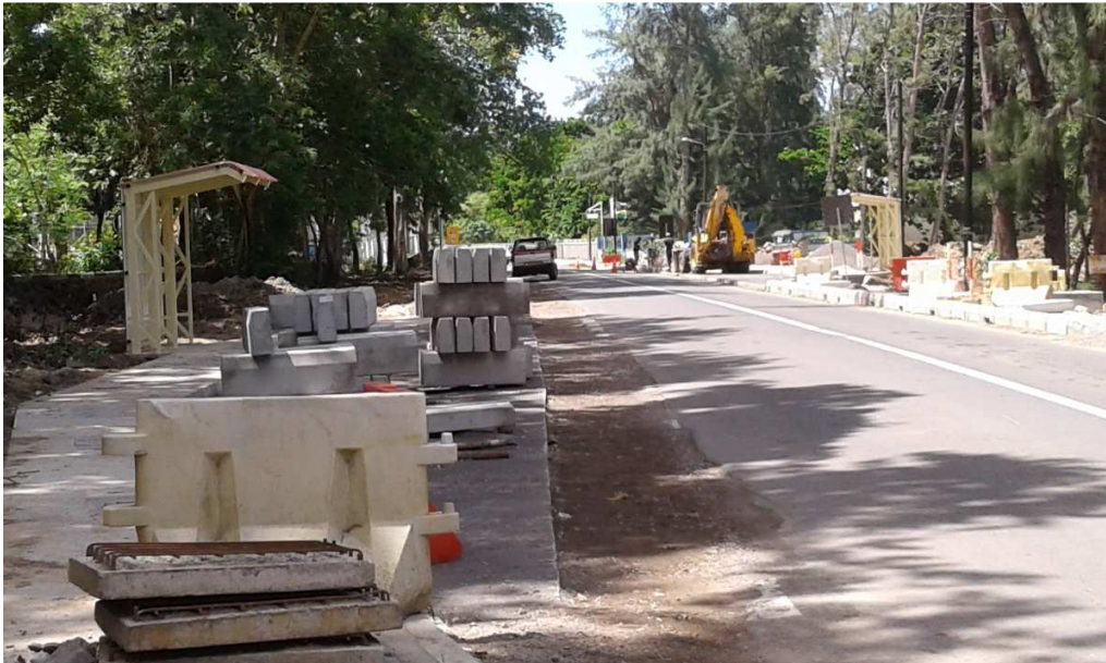
Figure 14: Two new bus laybys constructed with new bus shelters
