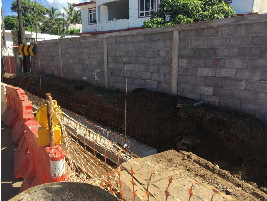
Figure 19: Laying of drain 500s at CH 315 to CH 335(ii)
