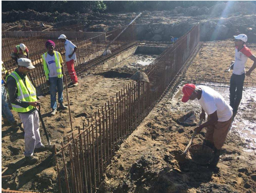
Figure 1: Backfilling, compacting and preparing platform of floor
