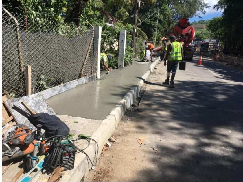
Figure 17: Casting of raised footpath
