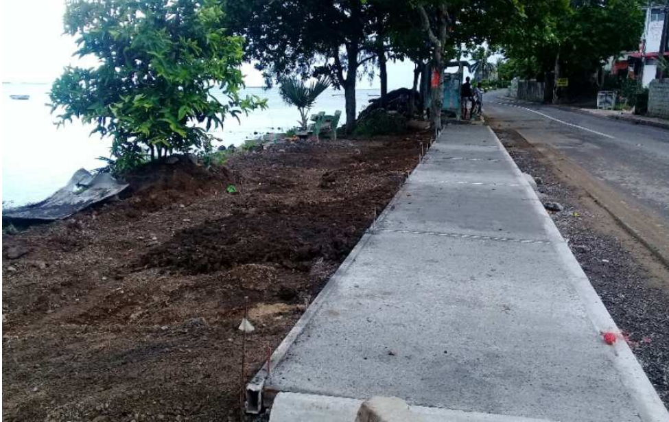
Figure 21: Casting of footpath
