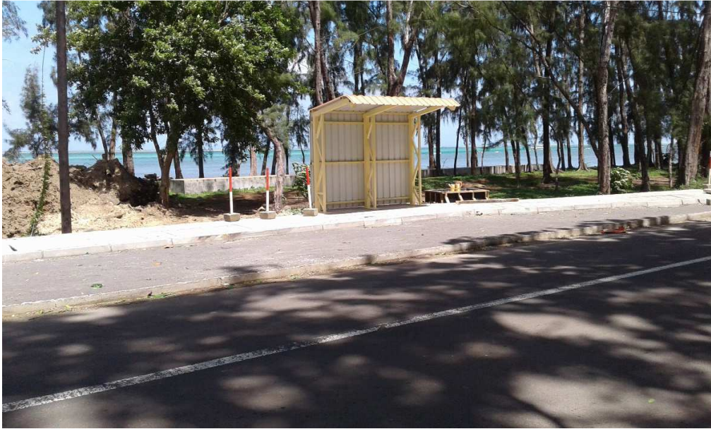
Figure 15: New Bus shelter placed
