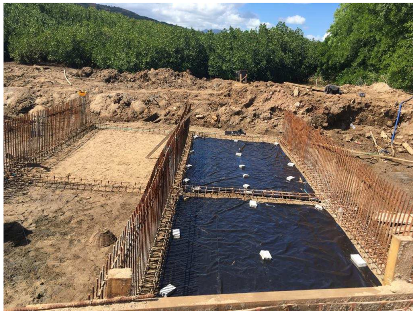
Figure 2: Preparation of platform for floor
