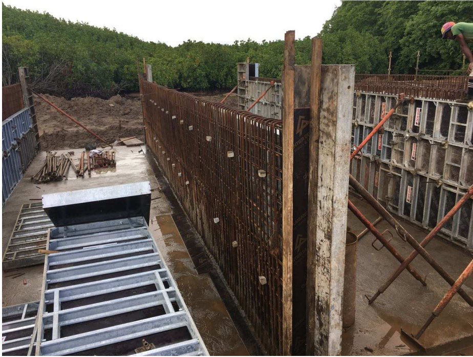
Figure 9: Preparation for shuttering
