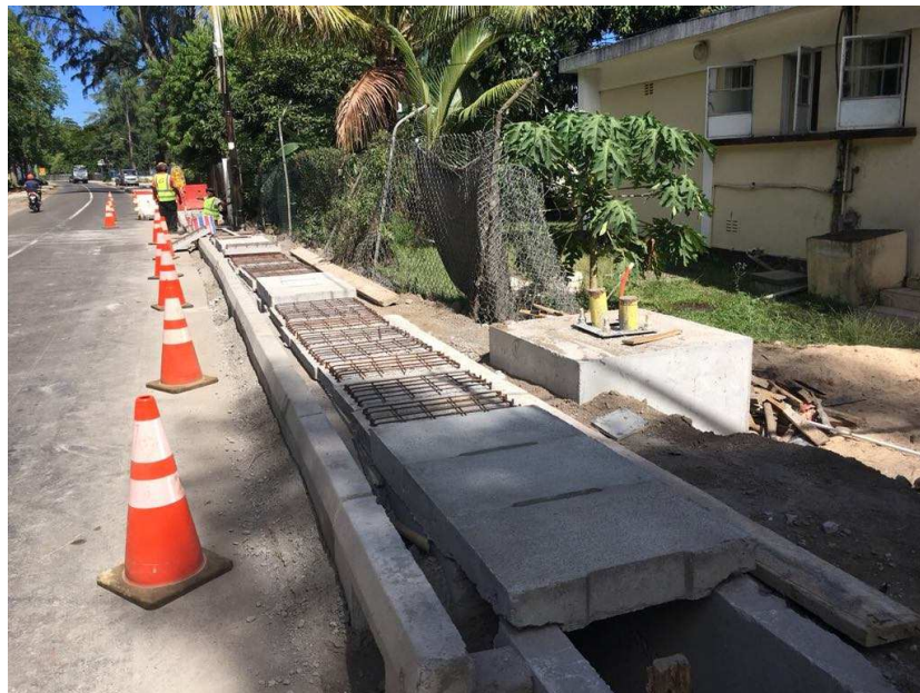
Figure 16: Raising of openable slabs and footpath
