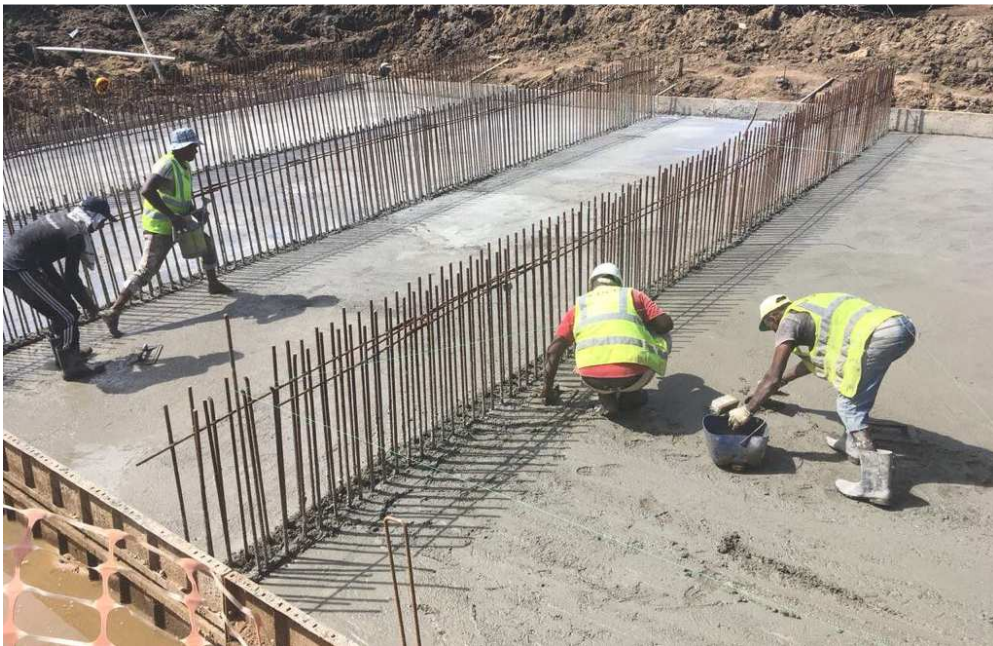
Figure 6: Finishing work on culvert floor
