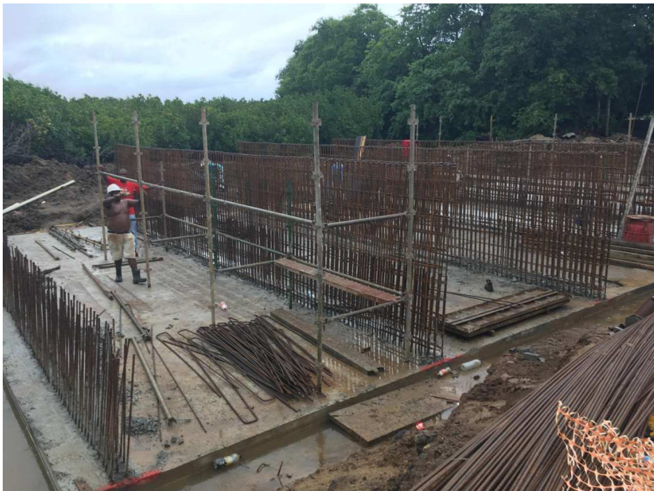
Figure 8: Erecting scaffolding for shuttering of wall
