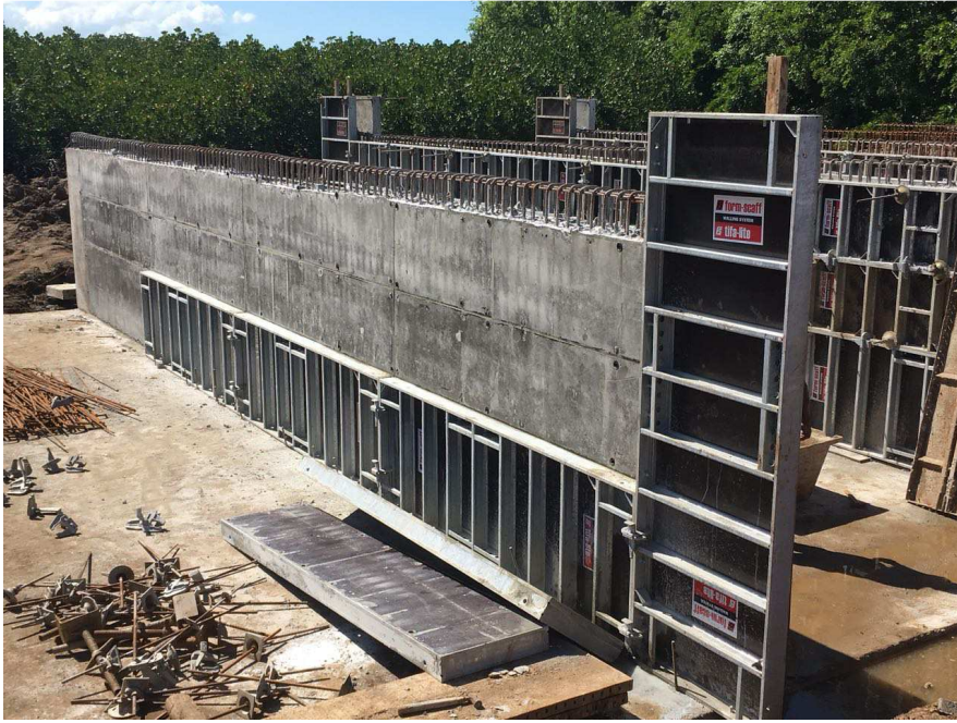
Figure 11: Culvert wall casted
