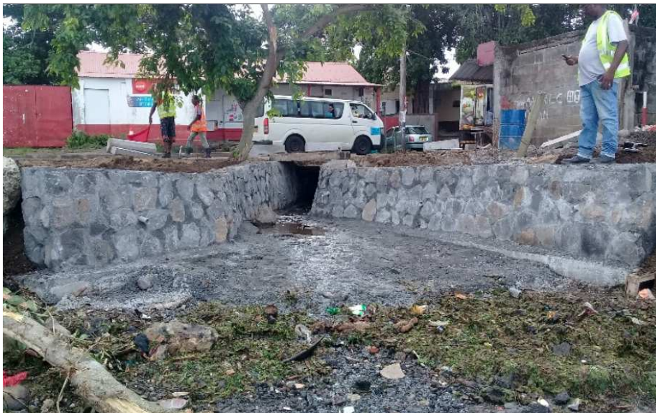
Figure 20: Construction of Masonry drain – CH 390.0
