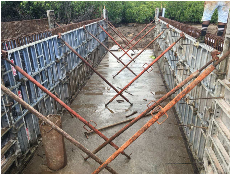
Figure 10: Shuttering of casting of culvert wall
