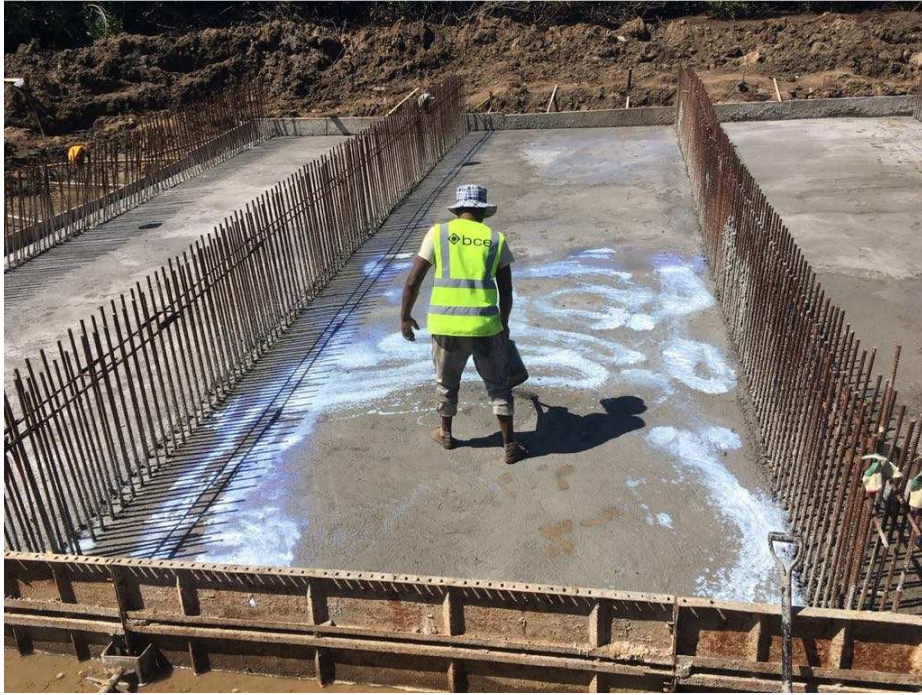
Figure 7: Spraying of Jetcure WB75 (curing compound)
