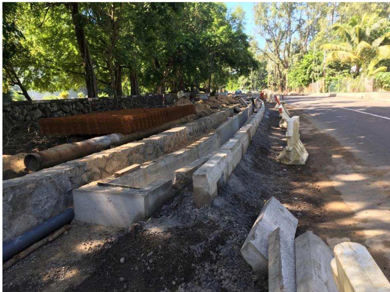
Figure 18: Laying of kerb at CH 130 CH 160
