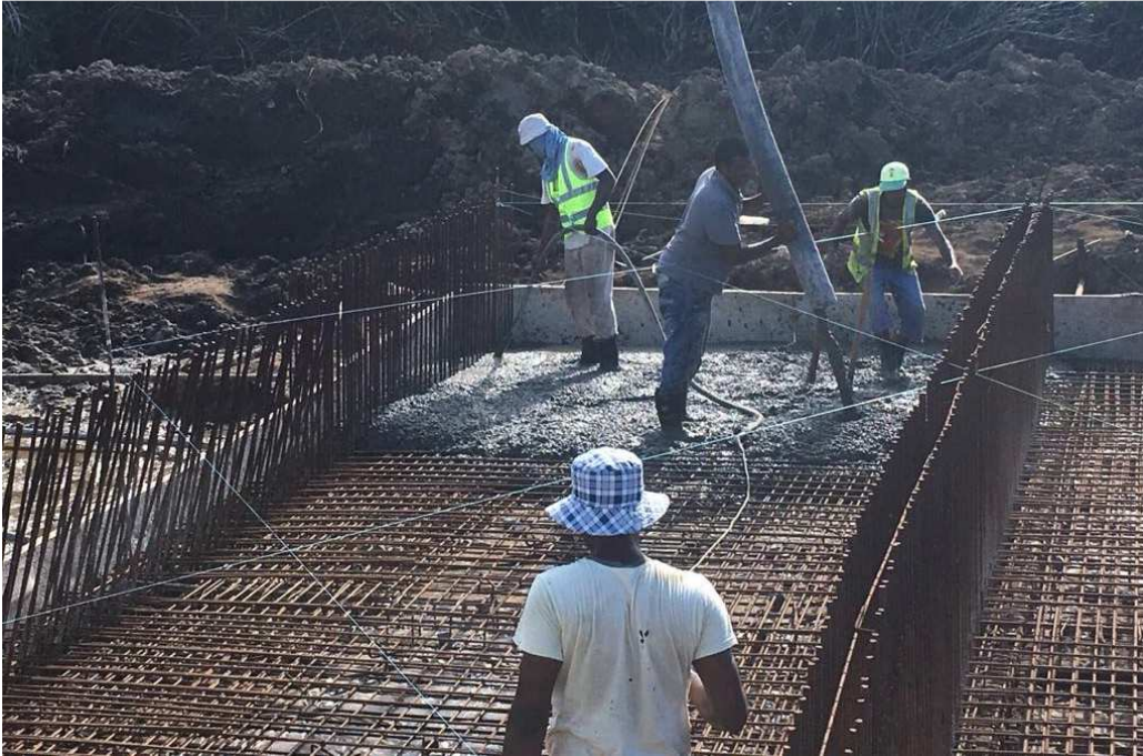
Figure 5: Casting of culvert floor
