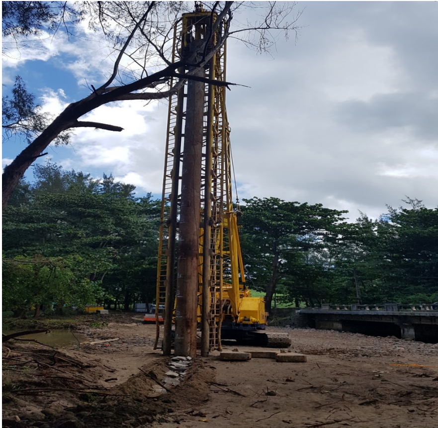
PILING WORKS ON SITE
