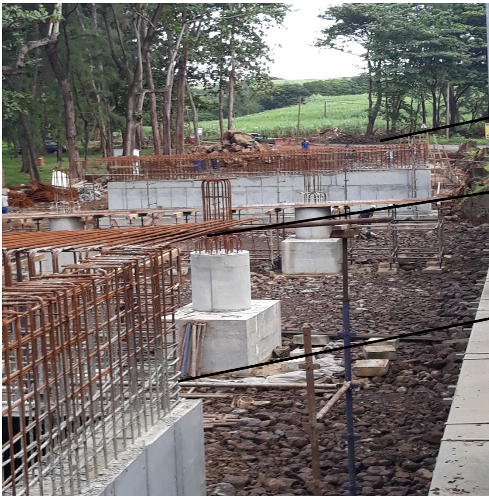
PILE CAPS BETWEEN ABUTMENTS
