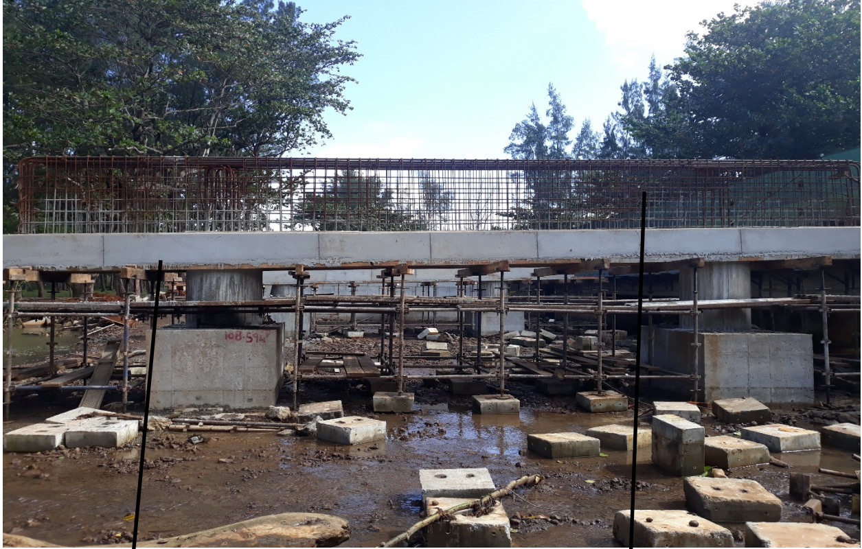
UPPER PART OF TRANSVERSE BEAM TO BE CASTED LATER WITH LONGITUDINAL BEAMS
