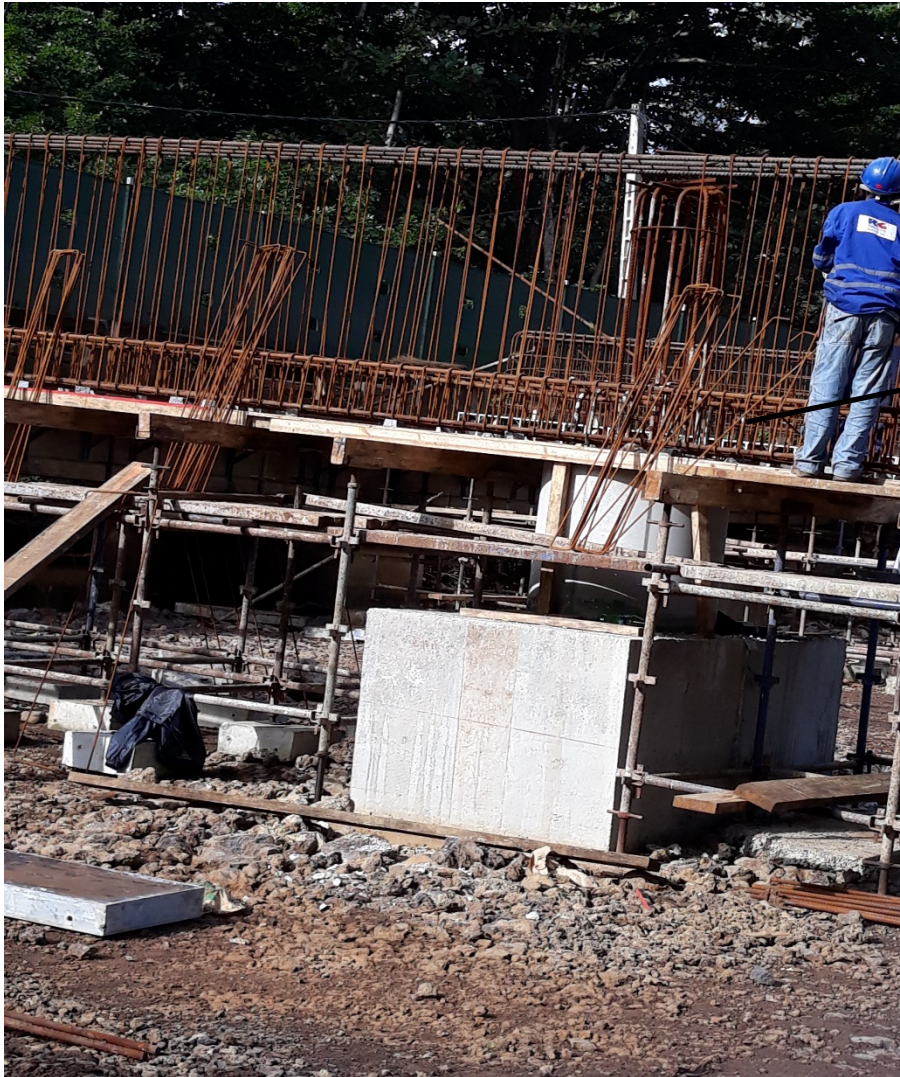
PLACING OF STEEL REINFORCEMENT FOR TRANSVERSE BEAMS
