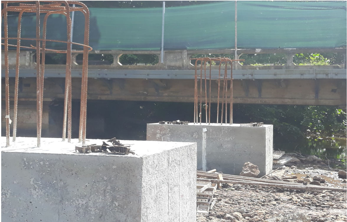
PILE CAPS BETWEEN ABUTMENTS
