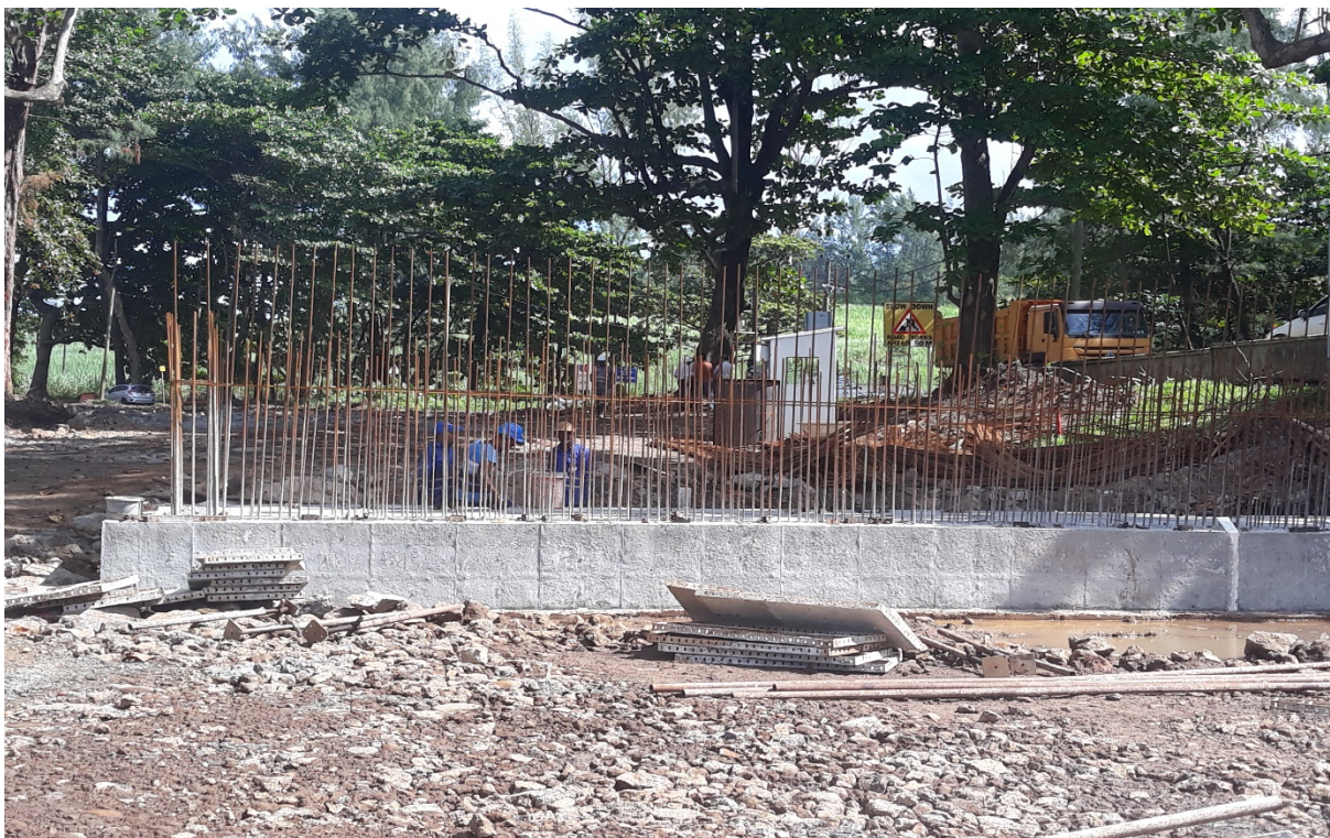
PLACING OF STEEL REINFORCEMENT FOR ABUTMENT WALL
