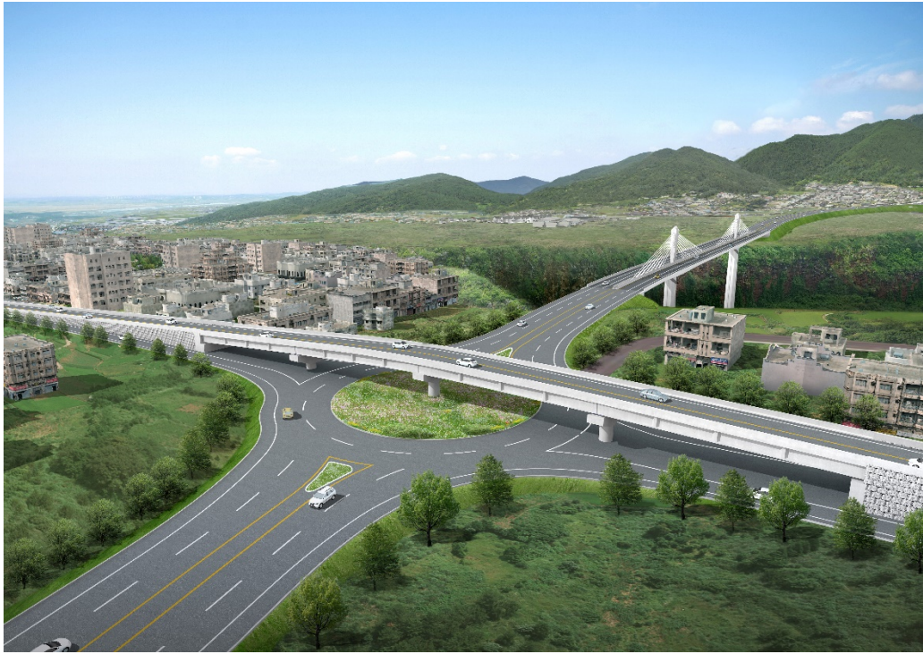
Plate 1: Chebel Viaduct and Roundabout
