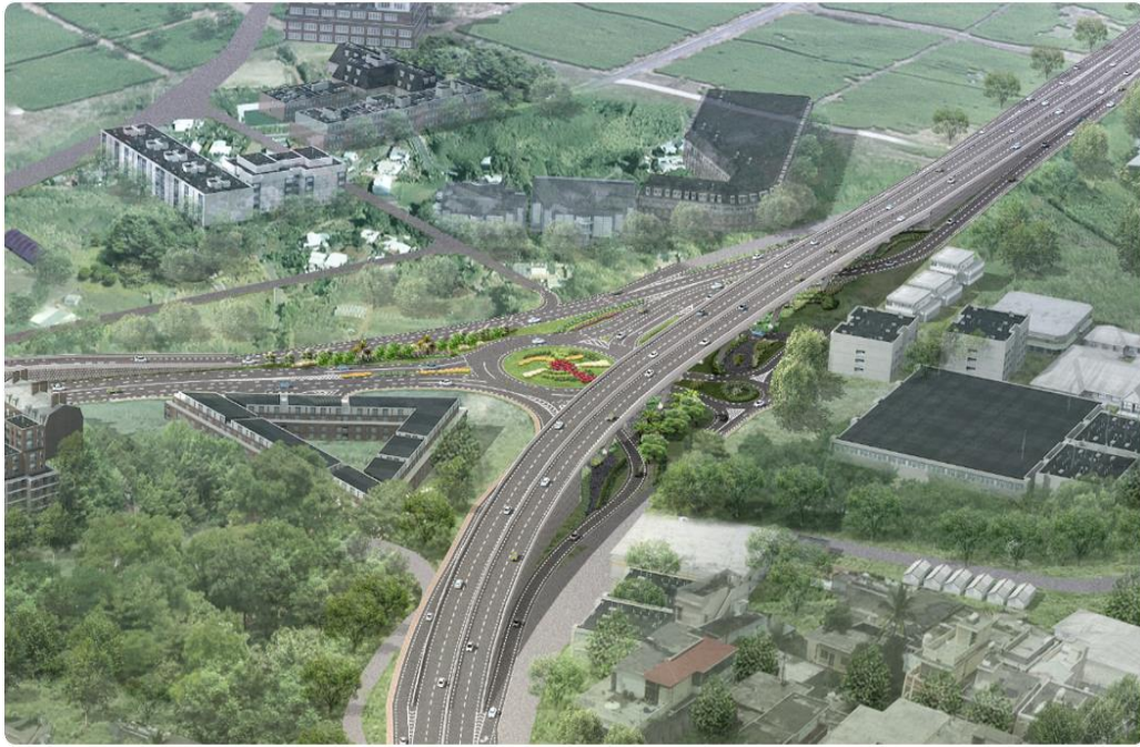
Plate 1: Grade Separated Junction at Pont Fer
