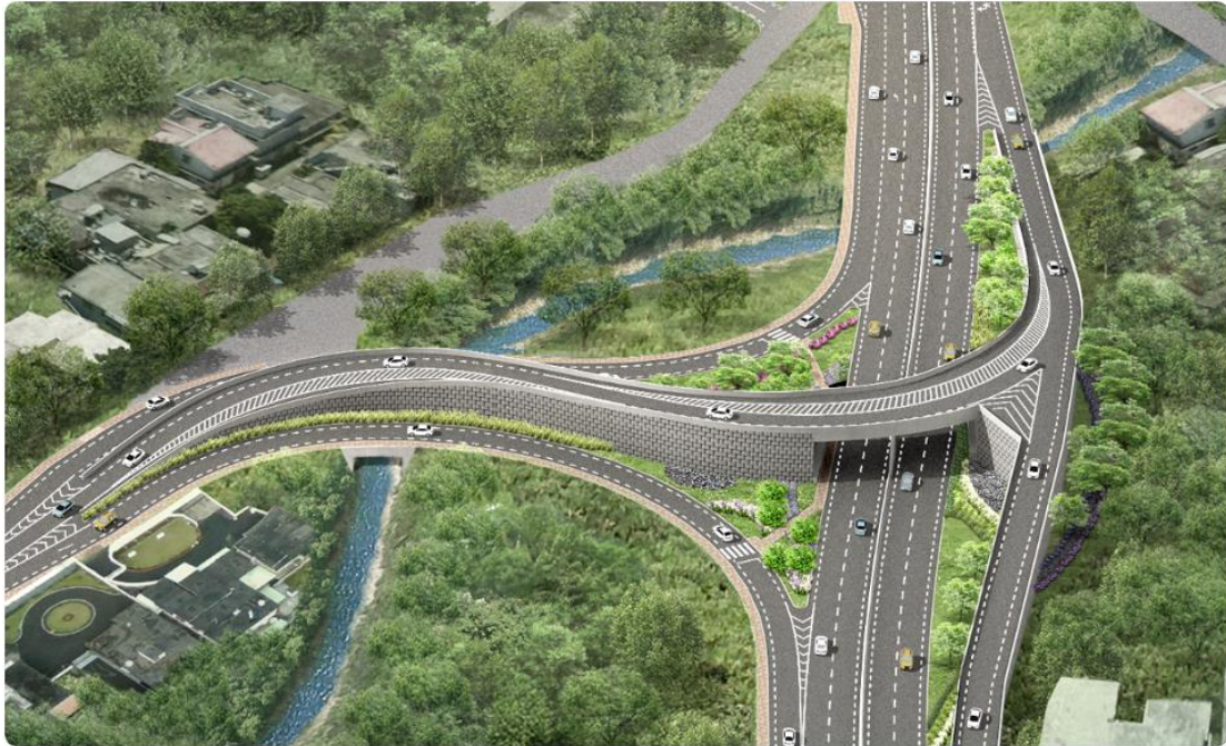
Plate 3: Grade Separated Junction at Dowlut
